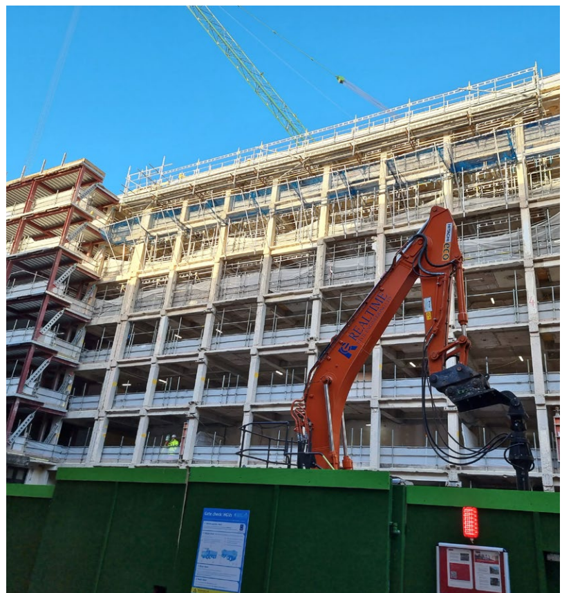
We jacked the entire hotel up whilst we excavated below before transferring its weight onto newly constructed foundations.
