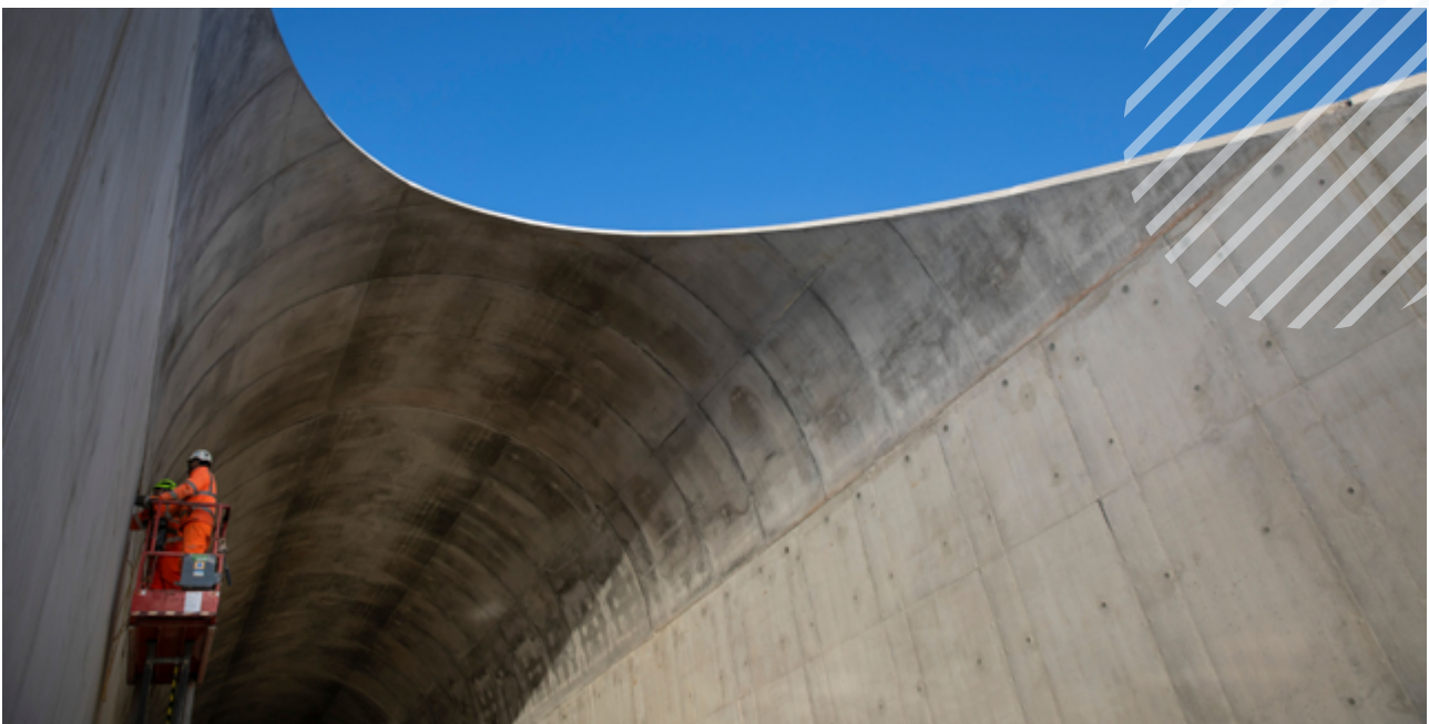
The mouth of one of the extensions designed to stop 'sonic boom'.
