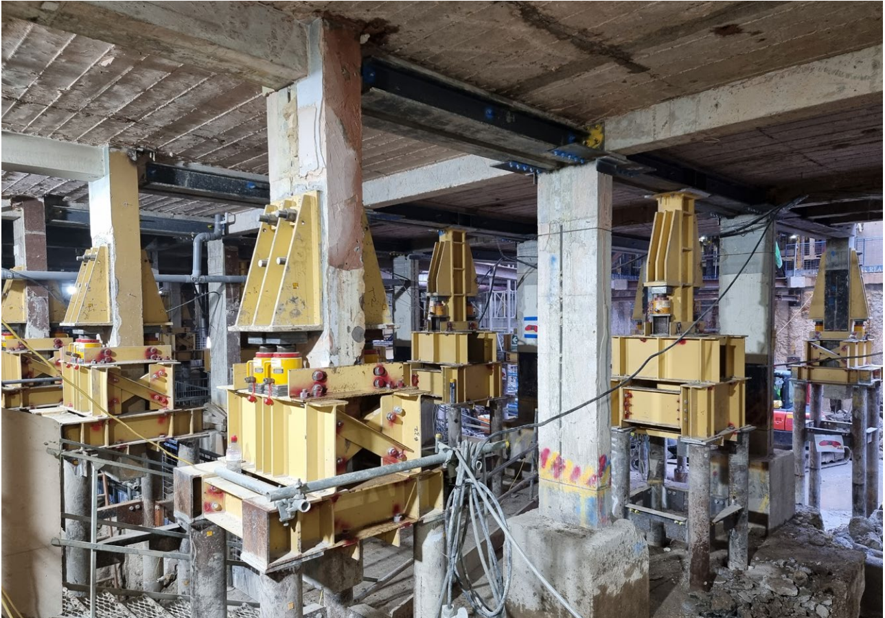
We jacked the entire hotel up whilst we excavated below before transferring its weight onto newly constructed foundations.
