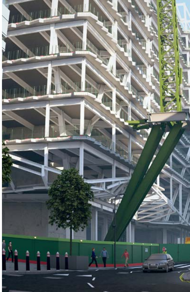
This render by our visualisation team shows how M 2 Alpine Lifting Solutions devised a solution where a crane that will be located 15m above a live highway is supported from the project's basement.
