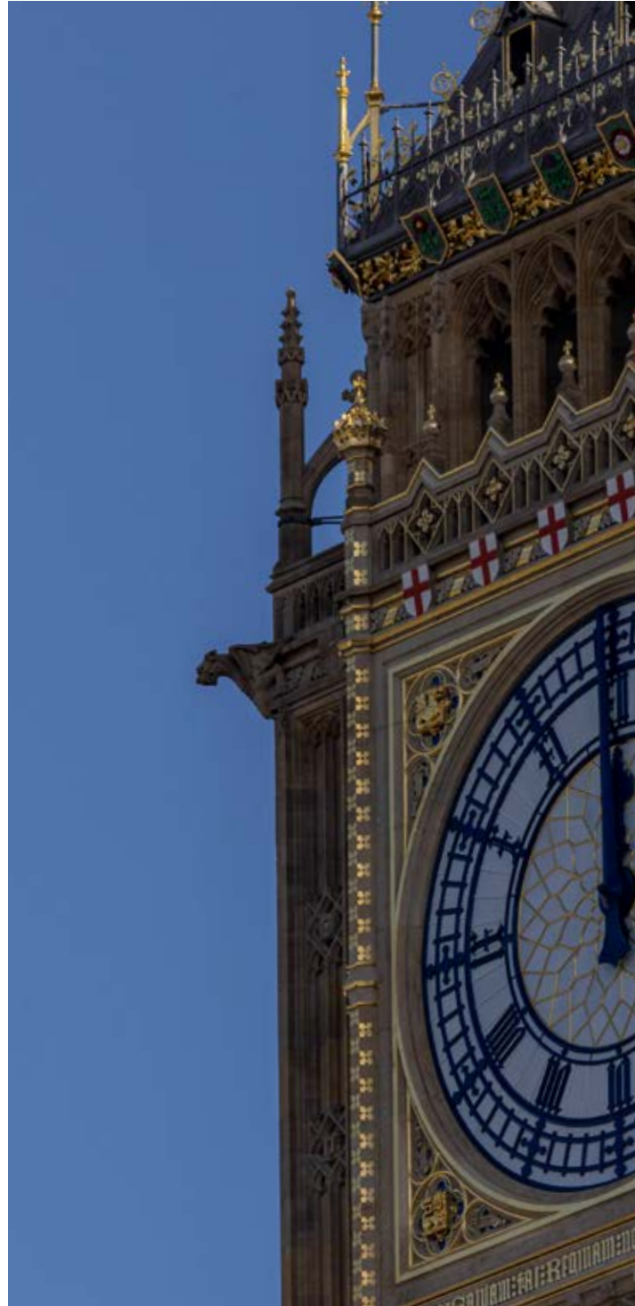
At Elizabeth Tower we have undertaken the largest repair and conservation programme in its rich history.
