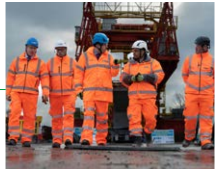
HS2 Minister Huw Merriman is the first person to walk along the Colne Valley Viaduct.
