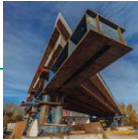
A533 Expressway bridge installed over the M56 in a weekend closure.
