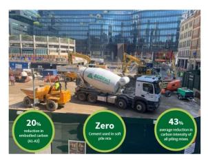
At 1 Broadgate, the team successfully increased the amount of GGBS content in the hard and soft piles to 70% and 95% GGBS respectively, with the soft pile mix a specially developed low carbon solution containing less 12.5 kg cement per m3 of concrete.
