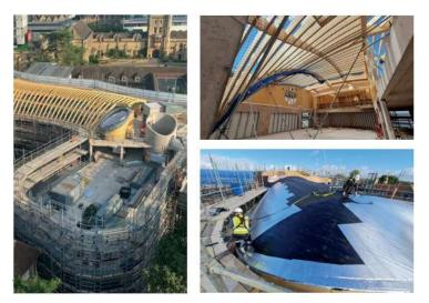
As part of a preconstruction services agreement with the client, we delivered a mock-up of the main quadrangle roof to explore construction techniques, temporary works, and the overall aesthetics. As a result, it was decided that the roof be redesigned. We therefore undertook a feasibility study exploring six alternative construction types and 15 different coverings with embodied carbon a key consideration for each option.
