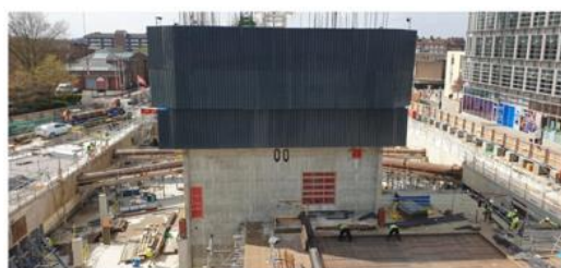
April '21 – Central core progressed up to level 2 – Ground floor construction started
