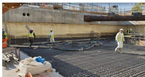
April '21 – Basement raft construction completed
