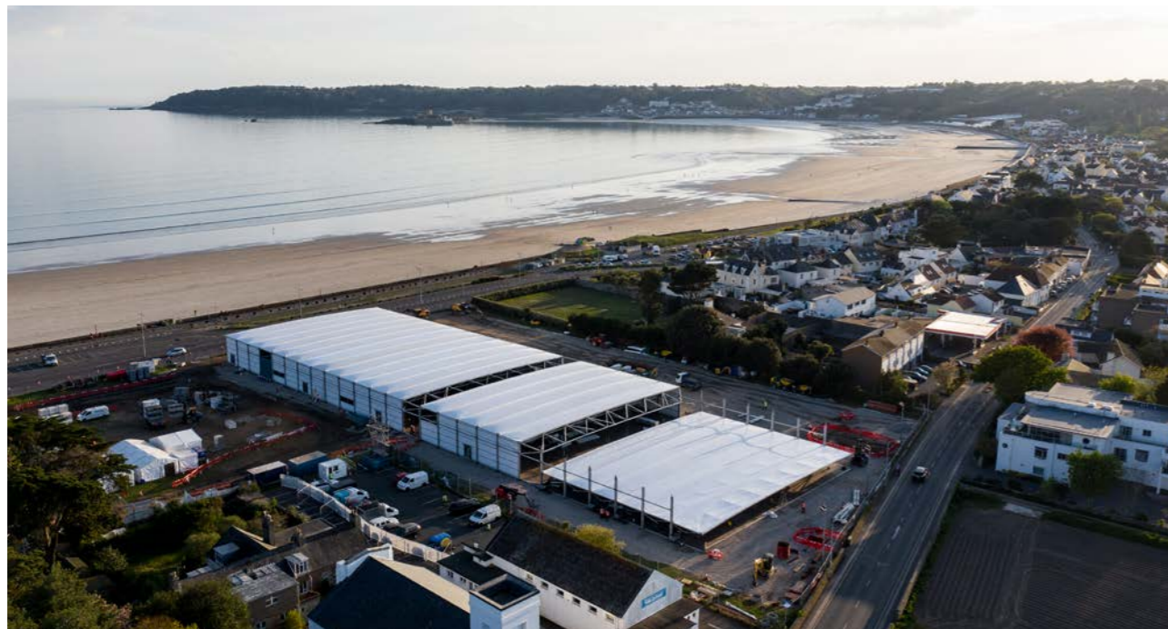
We constructed the Jersey Nightingale Hospital in just four weeks
